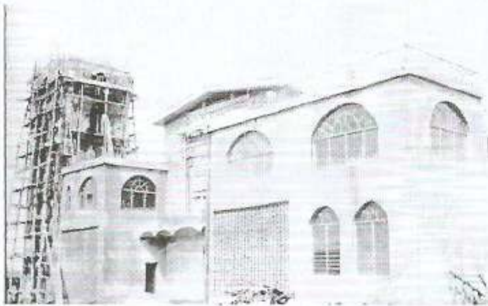
New Church under construction
