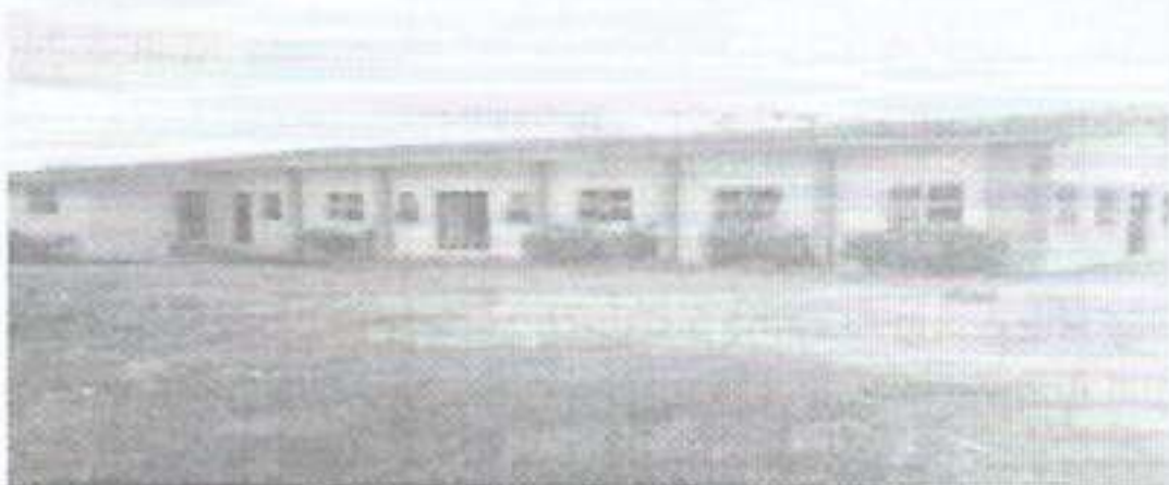
HOLY TRINITY ANGLICAN CHURCH, OKE-ARO, AKURE
