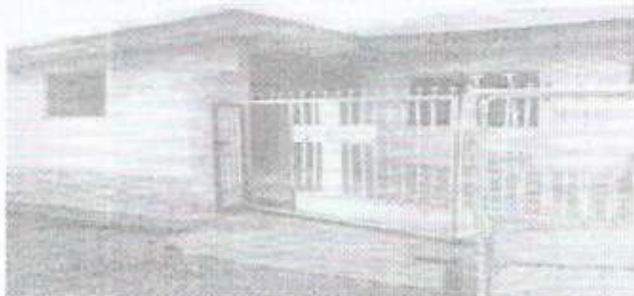
St. Thomas's Church Crèche foundation laid on 02-12-2009 and dedicated on 11-09-2011
