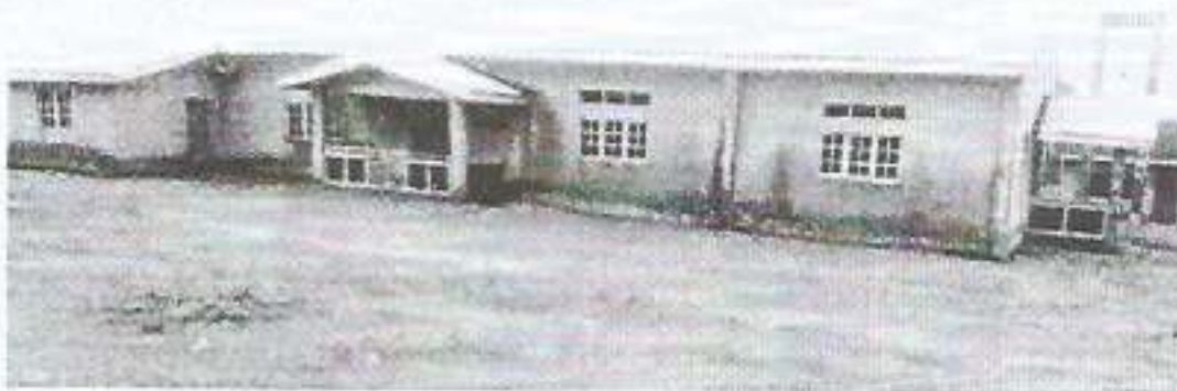
AKIN OMOSEEBI ANGLICAN CHURCH, ONDO ROAD, AKURE
