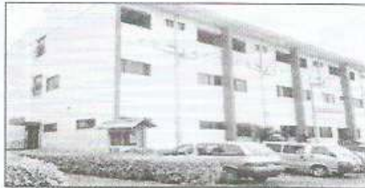
St. Thomas's Church Hall & Christian Education Centre on 3 Floors now been used as Offices, Priests Residences and Education Unit. Foundation laid 30th Sept., 1999 and dedicated 7th July, 2005
