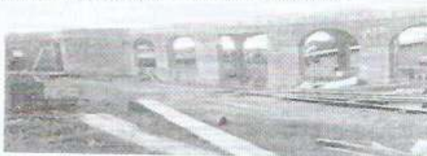
ISOKO / URHOBO ANGLICAN CHURCH, AKURE, UNDER CONSTRUCTION
